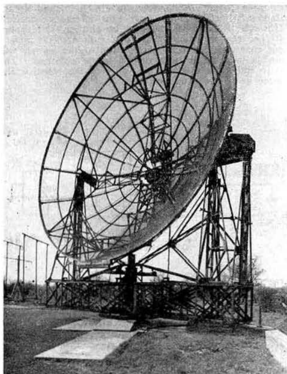
A 30ft steerable paraboloid for hydrogen line measurements on 21 cm. Note the fine mesh of the bowl and diminutive aerial at the focus. The Yagis in the background (left) are used for meteor echo techniques.
